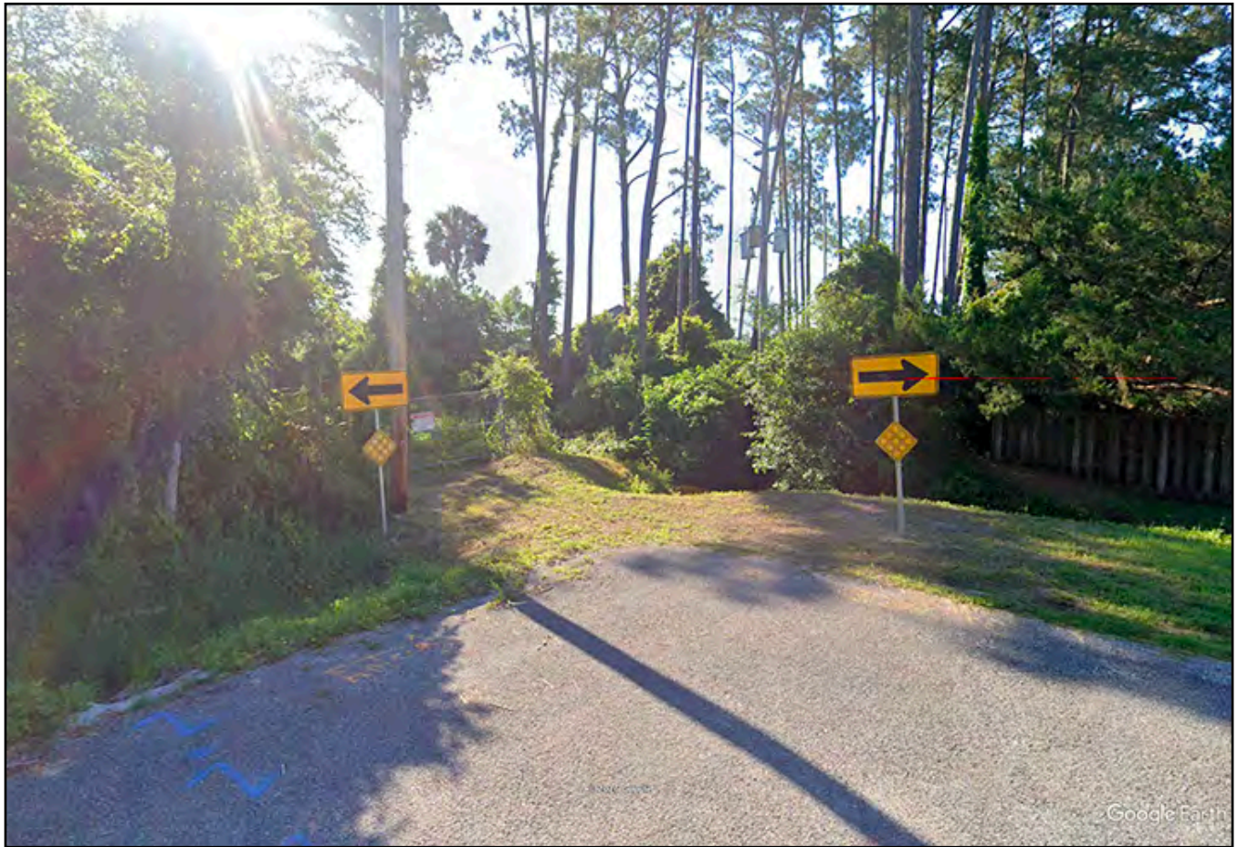
Figure No. 2 - Ditch termination point located at the intersection of Sixth Ave. and Ocean Blvd.
